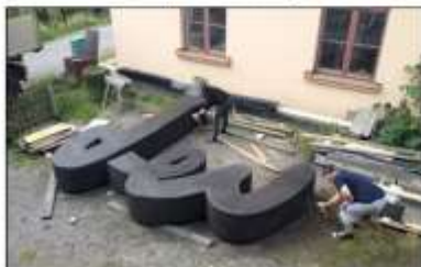
Bench LEV! Cement, heated and illuminated from below, 5m x 7.5m placed as the meeting point of the new train station.
