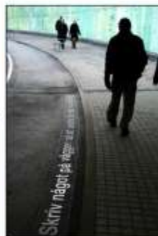
Quotes in bicycle path stainless steel in cement installed in asphalt
